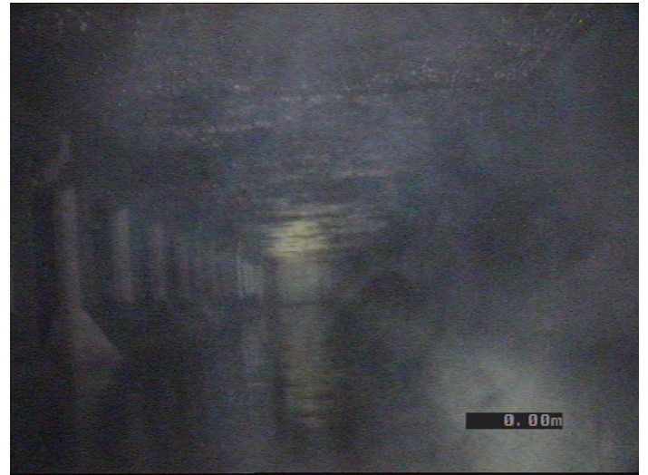
Start node type, manhole, reference MH1
