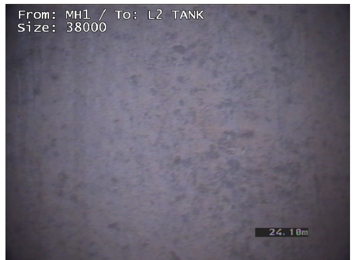
Manhole Finish (L2 TANK)
