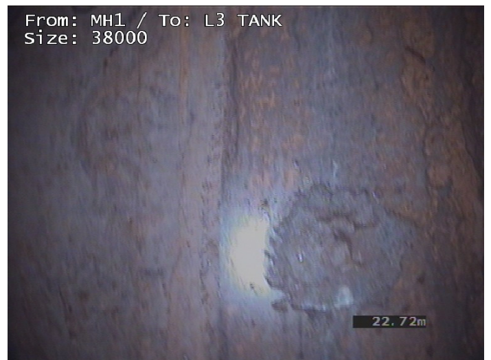
Manhole Finish (L3 TANK)
