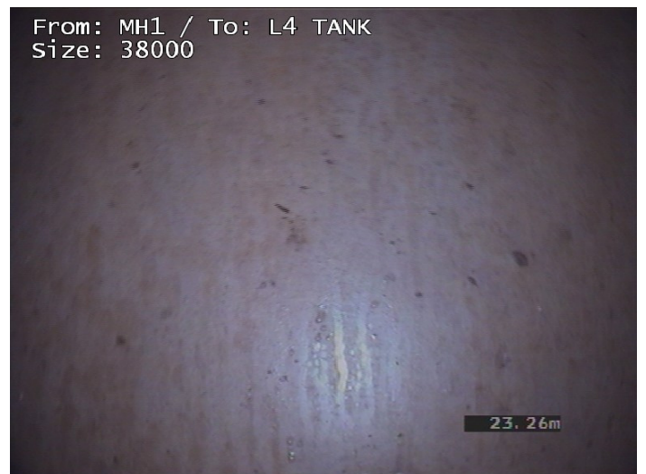
Manhole Finish (L4 TANK)
