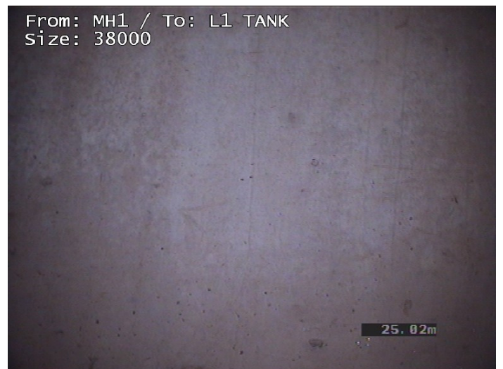
Manhole Finish (L1 TANK)
